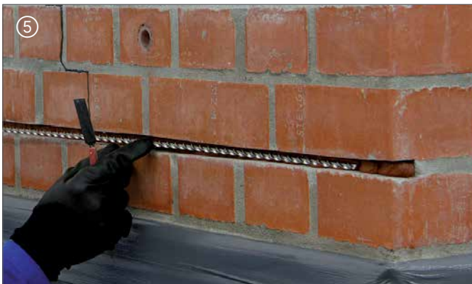
Spiralanker setzen | Place the spiral anchor
