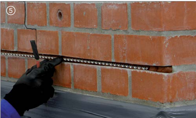
⑤ Spiralanker setzen | Place the spiral anchor
