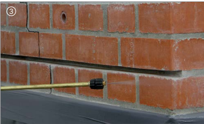
③ Fuge vornässen | Wet the joint / slot
