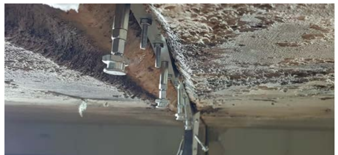
Eingebautes DESOI Quick Seal in einer Fuge | Built in DESOI Quick Seal in a joint
