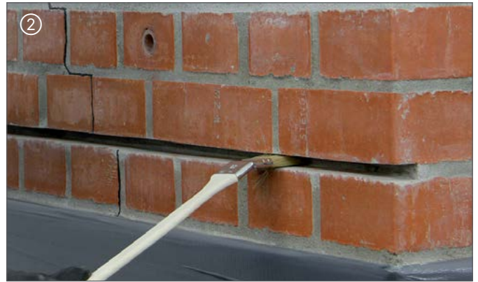
② Fuge reinigen | Clean the joint / slot
